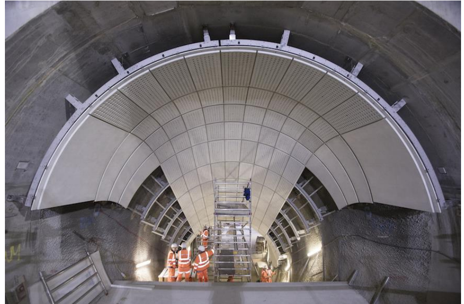
Photo: Bond Street Station Construction, Google Images.
